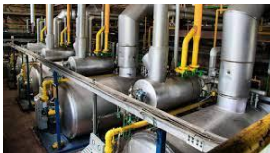
Figure 1.18 Regenerative Burners
