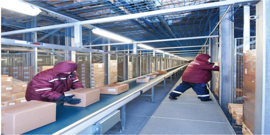
Fig 6.2 Automated Storage and Retrieval Systems
