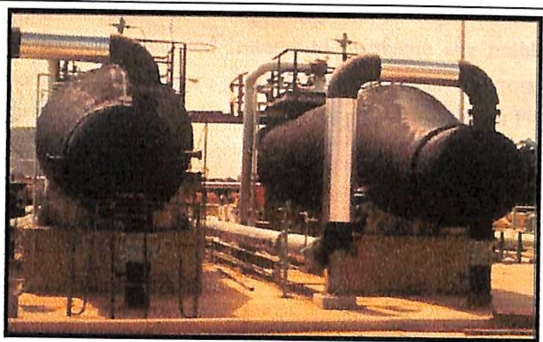
Figure 6.12: – Cove Point Vaporisers Source: Cove Point terminal U.S.
