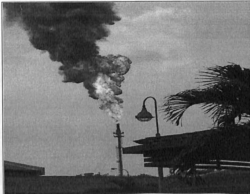
Fig.2.1: Gas flare at Star Refinery, Map Ta Phut, Thailand (Courtesy: http://en.wikipedia.org/wiki/Gas_flare )
