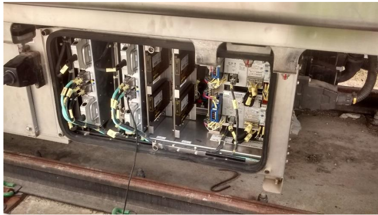
Figure 6: Propulsion Control Electronics System
