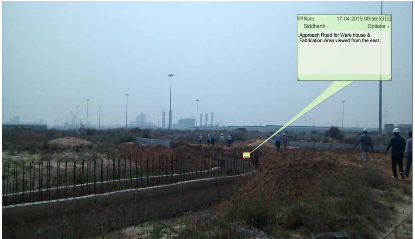
Figure 5.4: Approach Road for Warehouse & Fabrication Area
