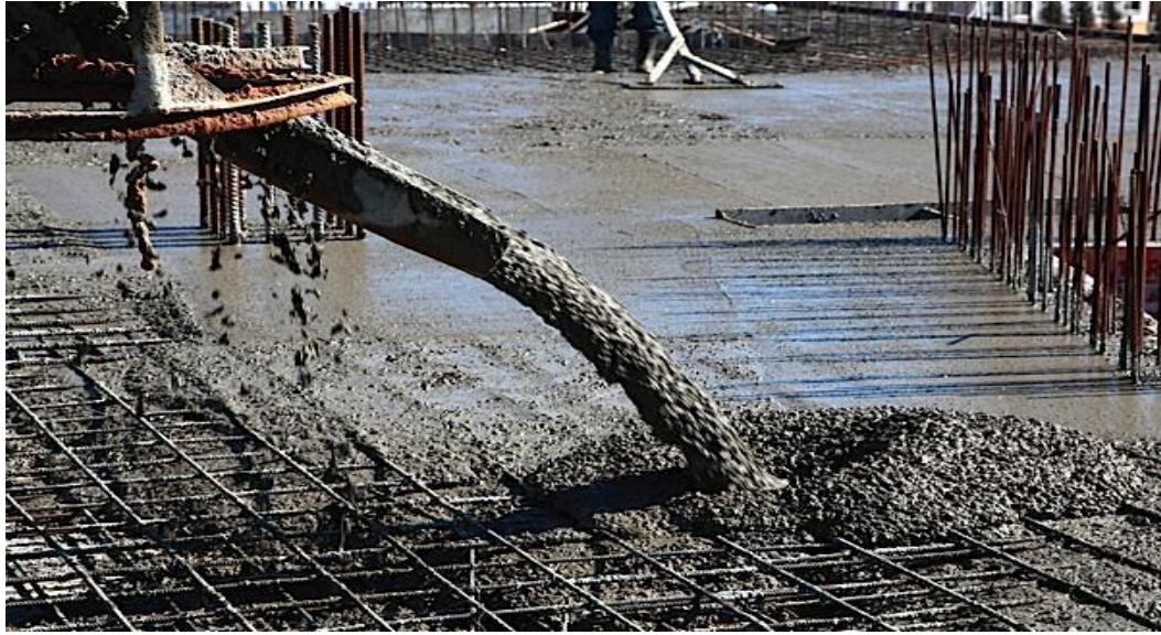
Figure 4.11 Plant Cement Concrete
