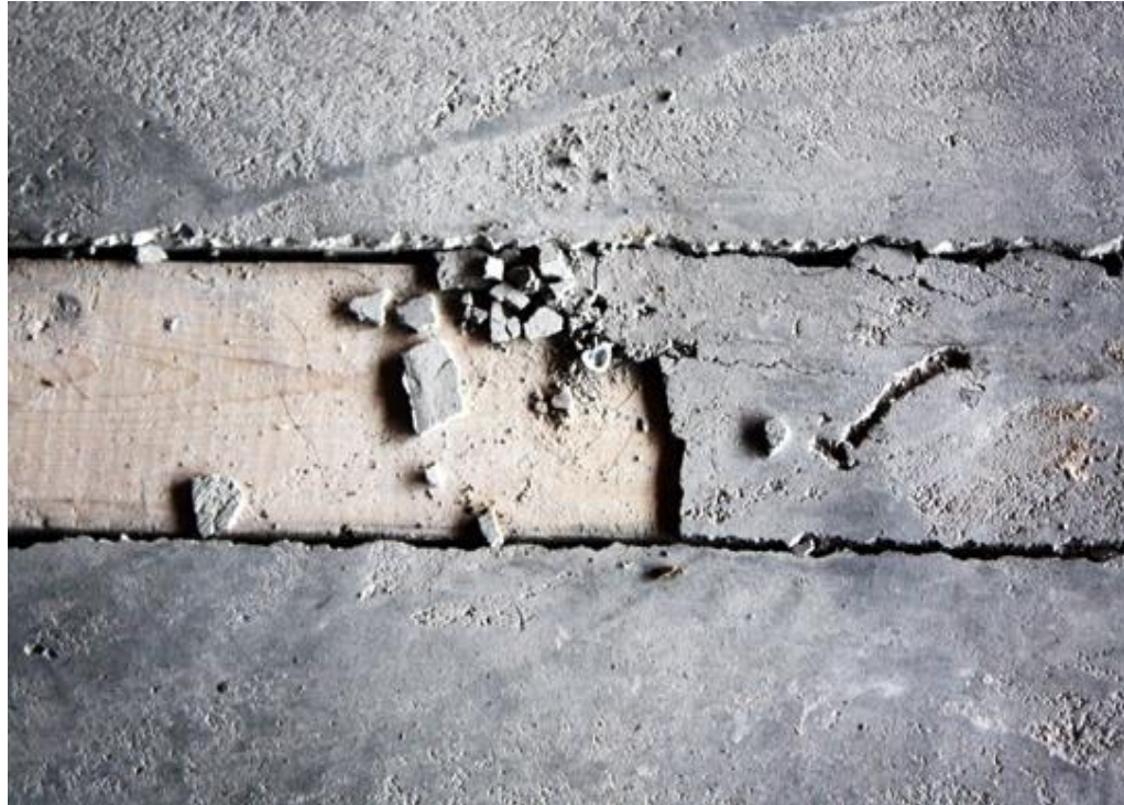
Figure 4.2 Chipping Work
