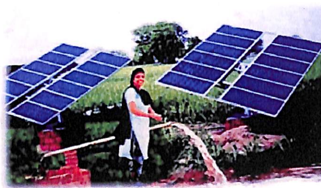
Figure 2.5: SPV pumping systems
