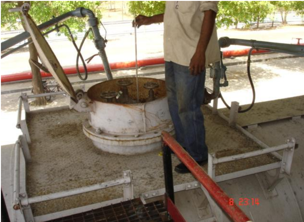
Figure12 – Rail wagon Loading activity
