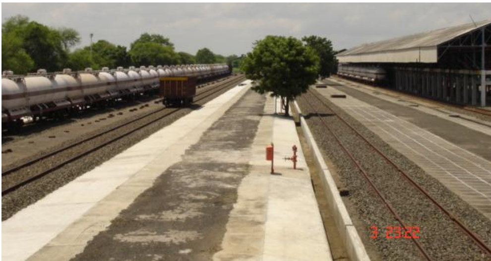
Figure 11 – Rail Loading Gantry
