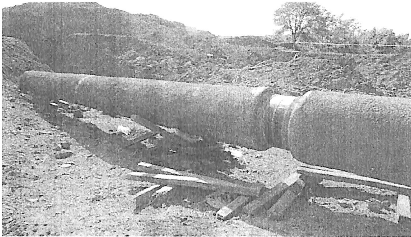
Fig: 9.2.2 Concrete coated Pipeline after welding
