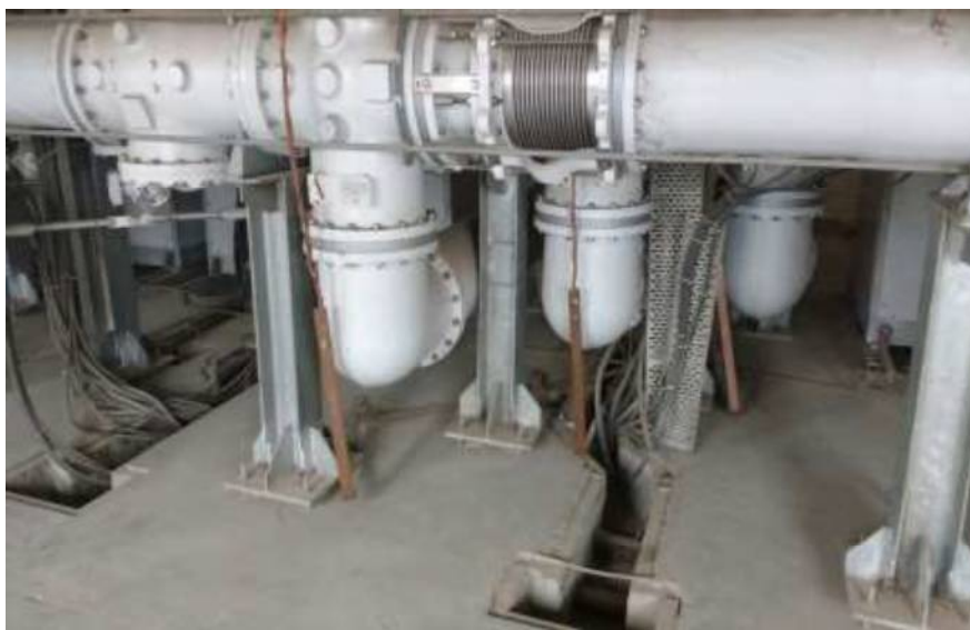
Fig 2.19 Grounding of GIS Enclosures-1
