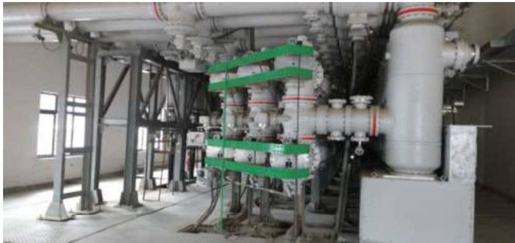
Fig 2.20 Grounding of GIS Enclosures -2
