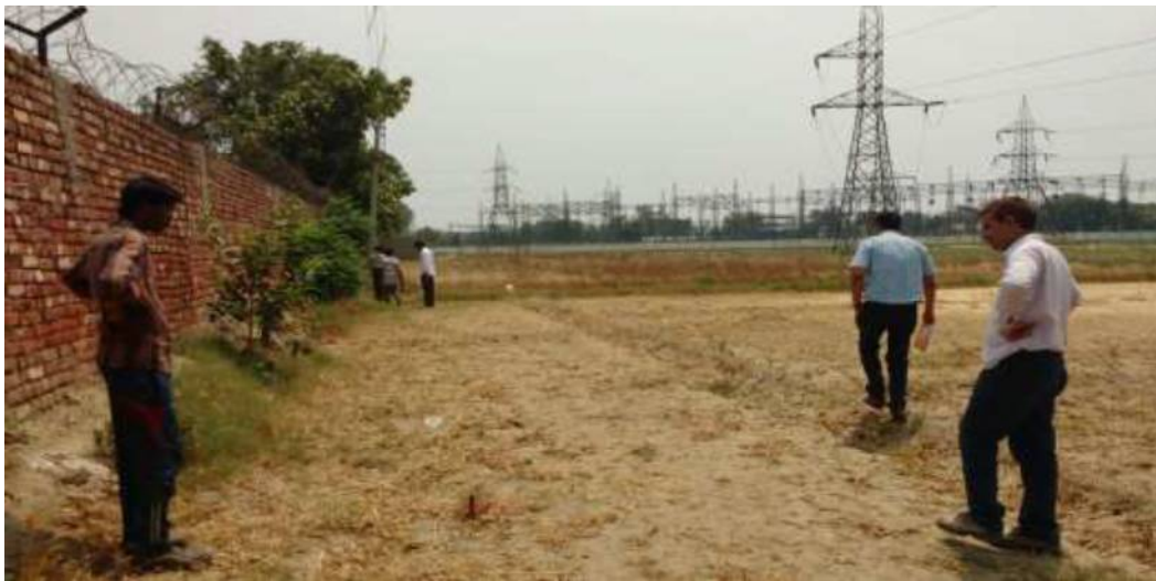
Fig 1.5 Resistivity Measurement in the Field (220 kV Narela)
