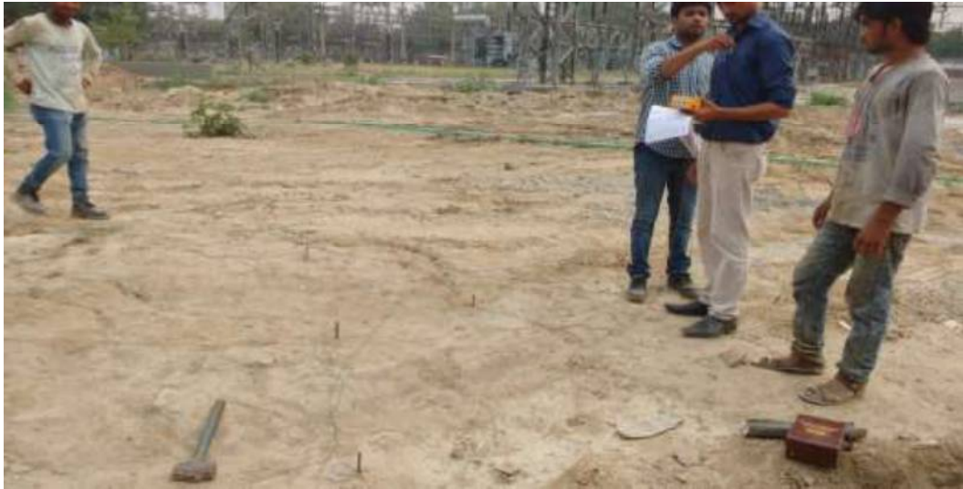
Fig 1.4 Resistivity Measurement in the Field ( 220 kV SMB)
