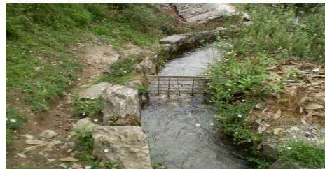
(Fig3.10:Wooden Screen at a site in Almora dated 29.06.2008 )
