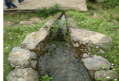
(Fig 3.5:Open penstock of a watermill at Chakrata dated 18.06.2008 )
