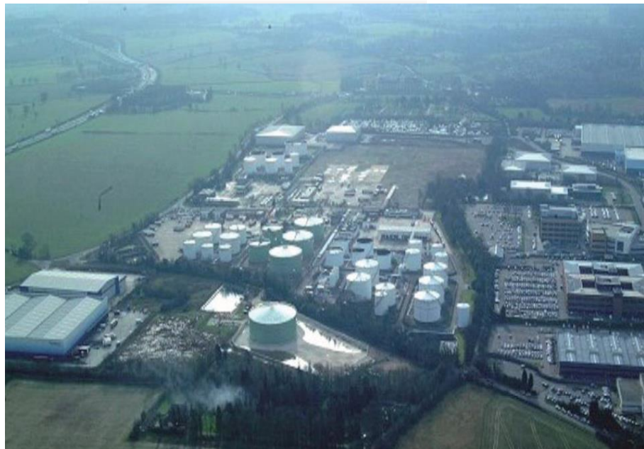
Figure 2.1 Aerial view of the Buncefield depot before the incident
