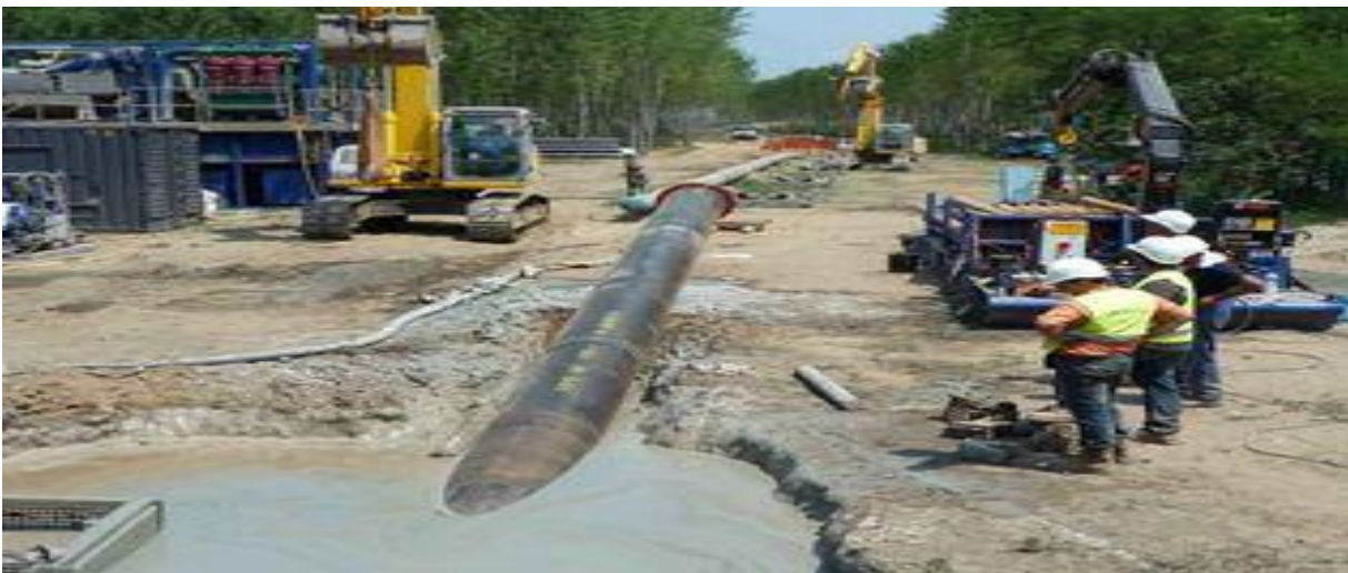
Fig source: apollotrenchless.com
