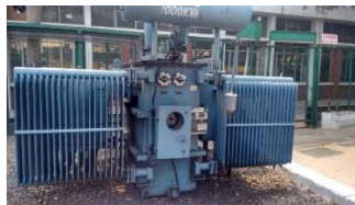
Fig 2.1 Transformer
