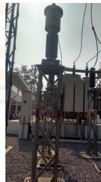
Fig 2.3 Lighting Arrester
