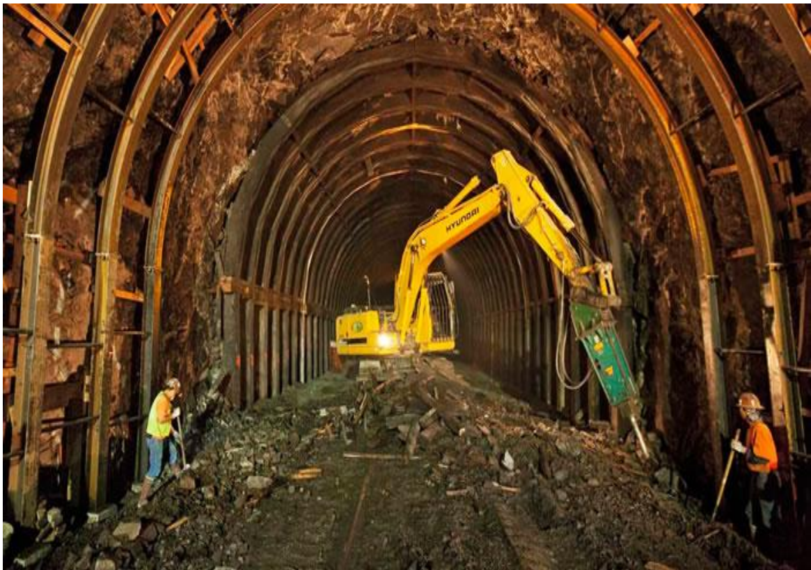
Figure.7: Steel Support System
