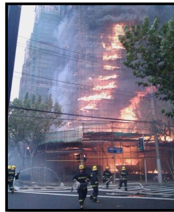
Fig.1.3: Shanghai building fire with combustible scaffolding platforms used for renovation work
