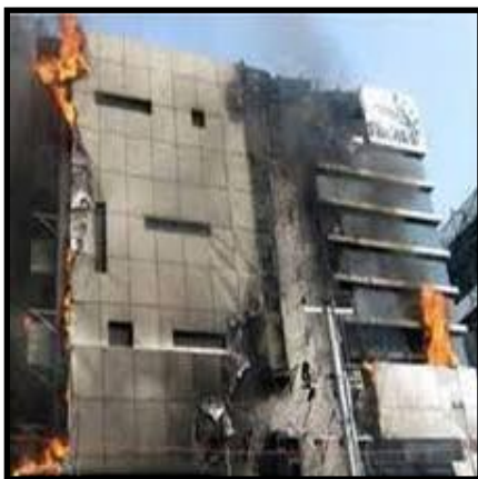
Fig.1.4: AMRI Hospital fire
