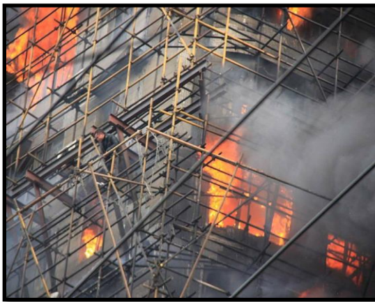
Fig.1.3: Shanghai building fire with combustible scaffolding platforms used for renovation work
