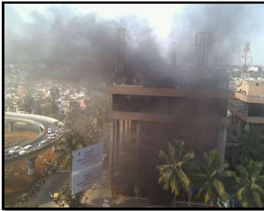
Fig.1.6: Fire at Carlton Towers, Bengaluru
