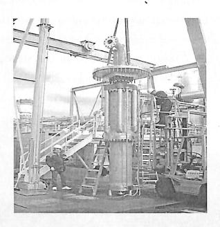
Fig-15 LNG Send out Pump
