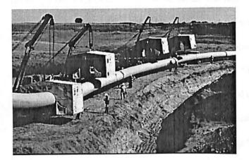
Figure 4: construction of X80 line pipe
