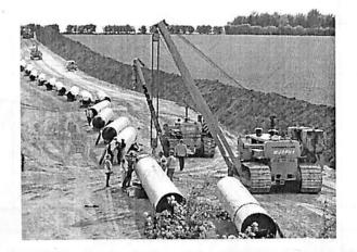
Figure 5: Transco X80 pipeline construction
