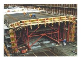
Figure 1.2: cut and cover method
