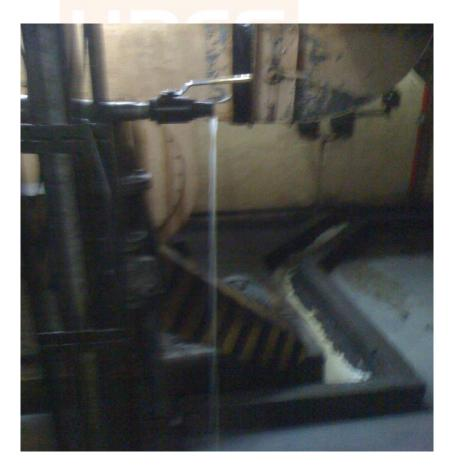
Fig 5: Leakage at Grinding Basement
