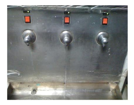
Fig 4: Leakage at Water Cooler
