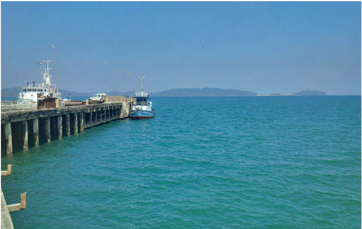
Figure 16 Arial Bay jetty in Diglipur
