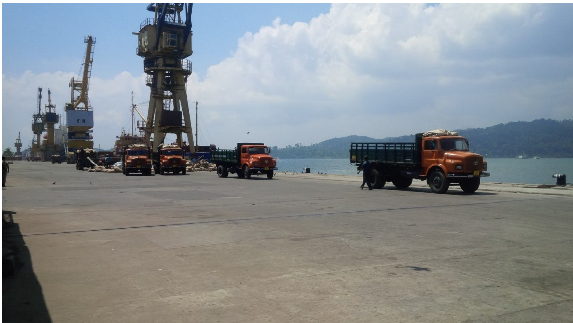
Figure 5 Haddo Wharf in the Port Blair Jetty
